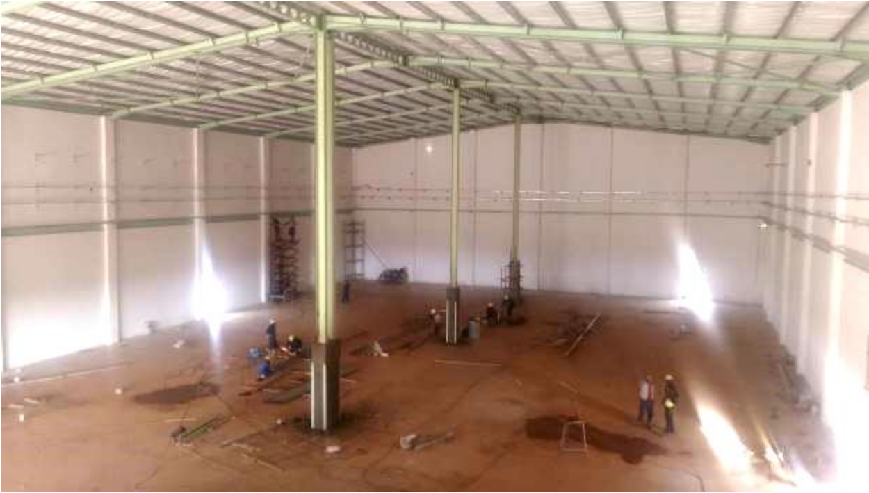
Figure2: Internal Wall Primer, 1 st Fix Plumbing & Electrical in ware house Building.
