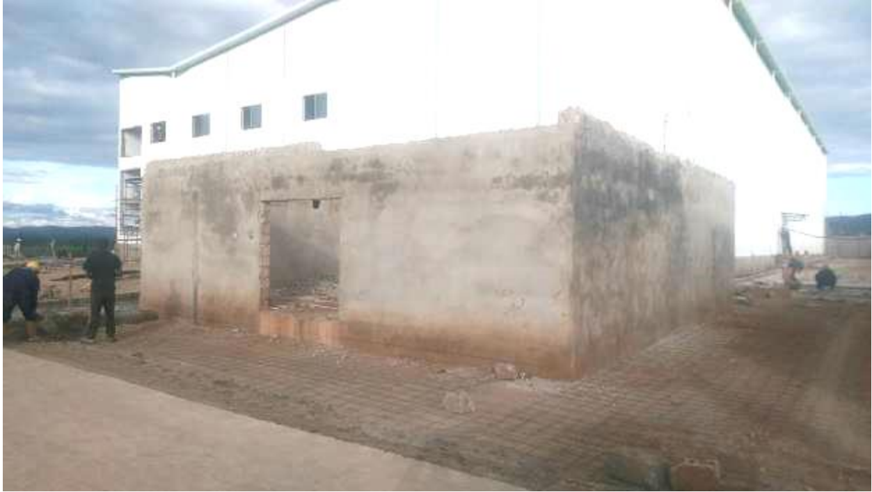
Figure 7: Front View of Demolished Hazardous Store Roof
