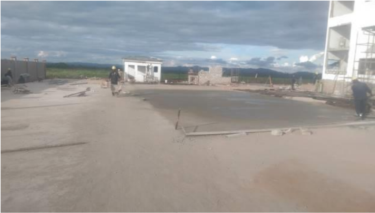
Figure 6: Concreting to the Driveway.
