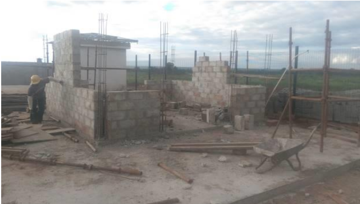
Figure 11: Construction of Lunch Shed Super-Structure
